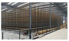
The assembly of the pallet racking for bulk storage is nearing completion. The racking, featured in the image above, comprises 35 aisles and will cover the majority of the warehouse floor space.
