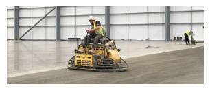
It is important that the floor is exactly flat. As manual picking will take place at up to 18 metres high, the slightest discrepancy at ground level could introduce significant deviation at that height.
