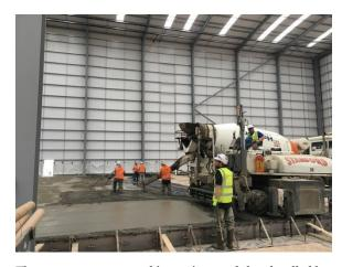
The concrete was poured in sections and then levelled by a topping spreader. Once each batch had set, the top was then levelled and smoothed by a machine that glides across the surface like a small hovercraft.
