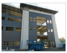
Following the completion of the roof and exterior walls, the warehouse is now weather-proof and this has allowed internal construction work to start.
