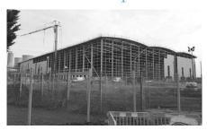
Following the completion of the main framework of the building, exterior cladding is currently being applied to create the outer walls and a roof.
